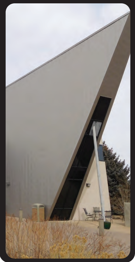
Colorado Welcome Center at Fort Collins (Photo by Tim Van Schmidt)
