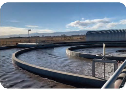
Wellington's wastewater plant (Photo courtesy of Town of Wellington)
